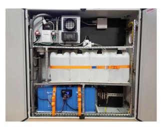
With a standalone battery solution with fuel cells a monitoring system of the client can be powered for a period longer than a month.
