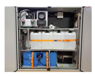
With a standalone battery solution with fuel cells a monitoring system of the client can be powered for a period longer than a month.
