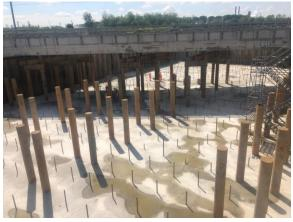
All anchors and piles were measured by divers when excavation-pit was full of water. When water was pumped out a total-station was used for a reference measurement. Result were spot-on and exactly the same.
