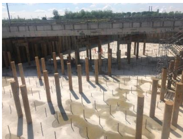
Excavation-pit, with GEWI-anchors and LEKA-piles
